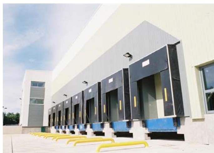
The new warehouse loading bays
