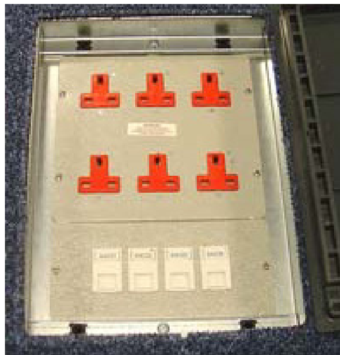
Floor box with LJ6C modules
